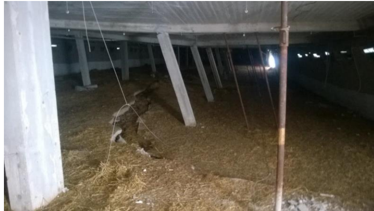
Figure: Examples of facility affected by landslide
